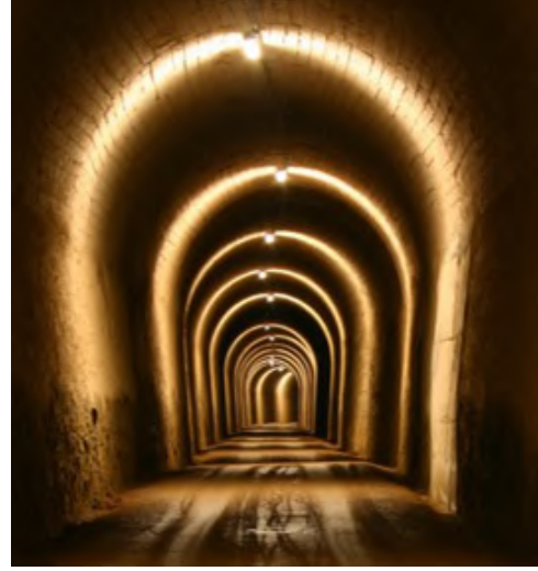
Fig. 2. View inside the Coripe tunnel. (Cadiz, Spain)
