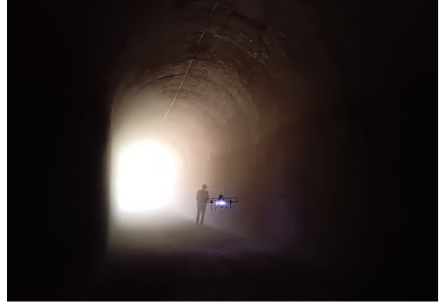
Fig. 1. Aerial robot performing a flight in a real tunnel environment.
