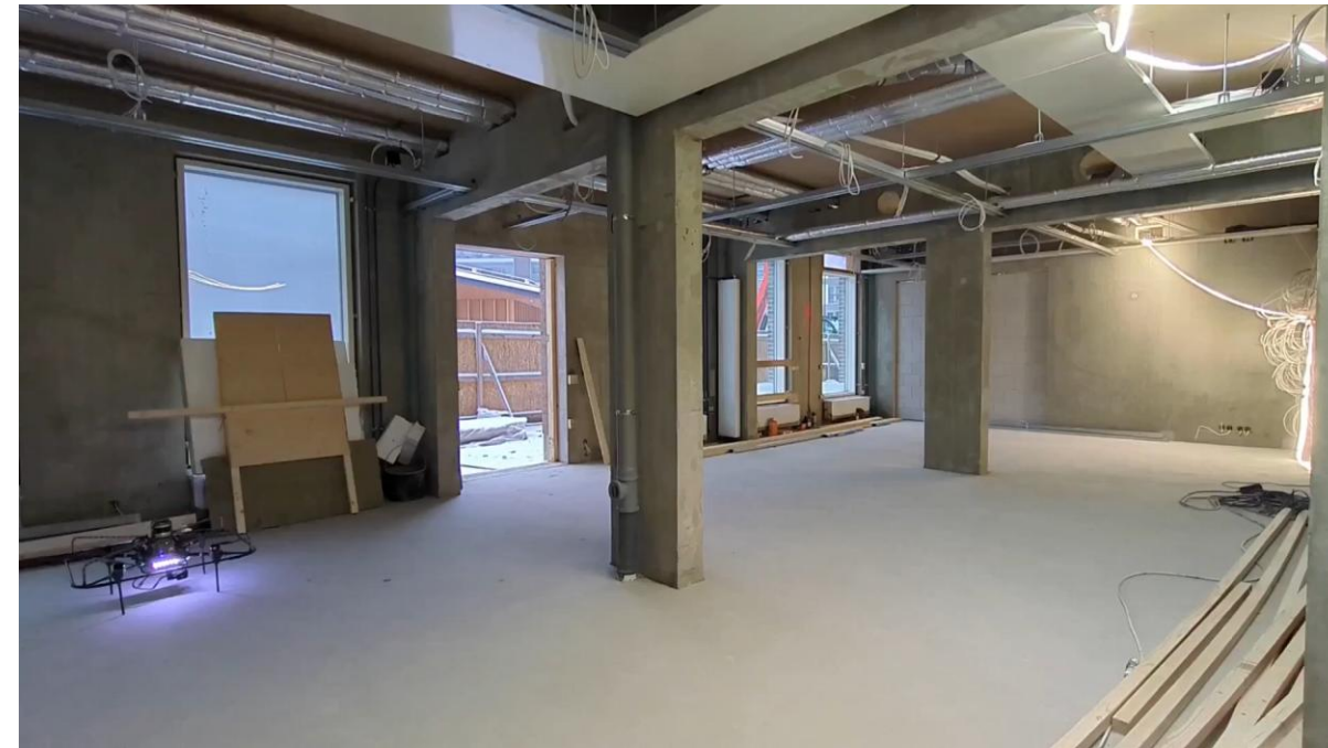
Autonomous mission execution – Outdoor Point-Of-View
