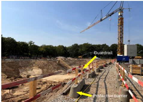
Figure 5: Installation of protective barrier to separate pedestrian worker walkway from vehicle traffic.
