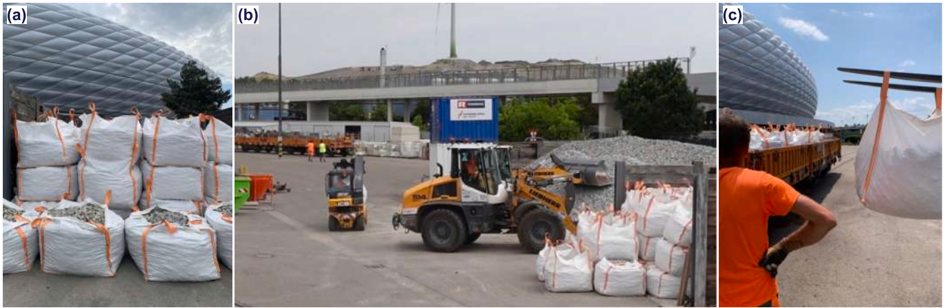
Fig. 7. (a) Railway ballast stored and waiting to be moved from the material staging zone to the railcars, (b) telehandler transporting ballast bags between the storage zone and designated waiting area for railcars, and (c) telehandler loading ballast bag onto the railcar for further transport, requiring pedestrian worker assistance in the loading and unloading process.
