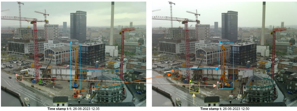
Figure 7. Detection and tracking of machines between two consecutive images
