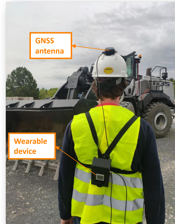
Road construction site
