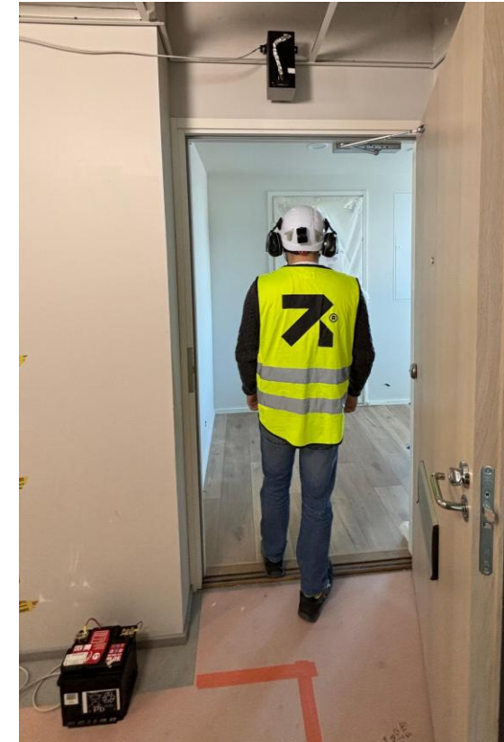
Building construction site
